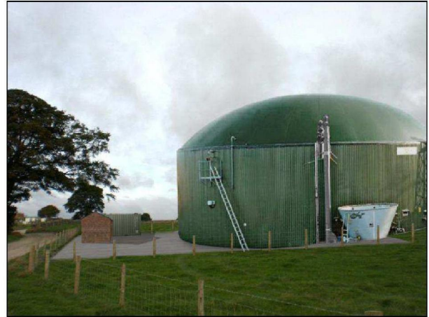
Figure 1 – Photo montage of a typical digester tank (Indicative Only)
